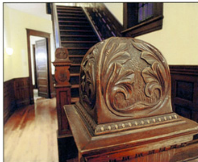
"A successful project is about communication, collaboration," Louis LaFratta said. Here, original woodwork on the first floor is preserved.
